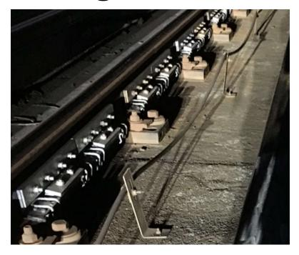
Same damper (400mm long) installed 1 or 2 dampers per metre of rail
