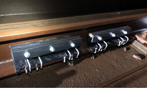
Two trial damper designs (300mm long) for areas with 500 mm fastener spacing
