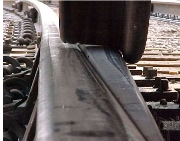
Switch point above stock rail
