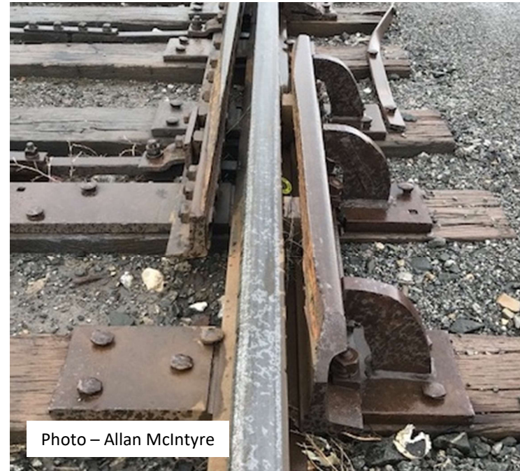
The Bethlehem design uses a machined piece of rail as the wear bar; it is not adjustable
