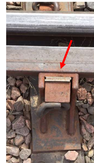
To adjust, move shims to shift guard rail inward
