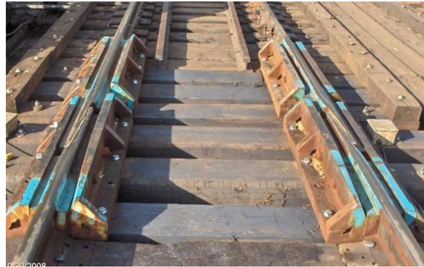
CTM uses tapered rail ends to support wheels across the joint. These rails also have a thick web, which creates a stiffer rail
