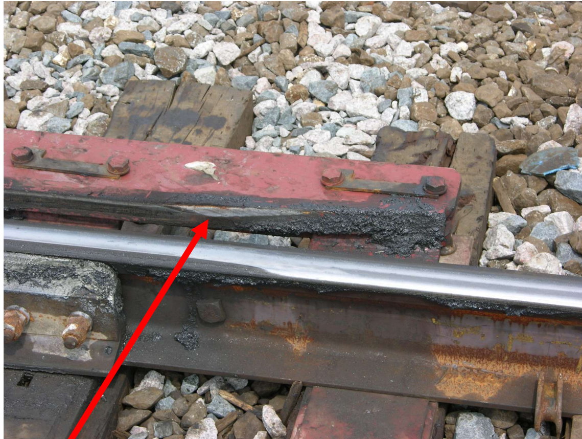
Heavy wear on switch point protector
