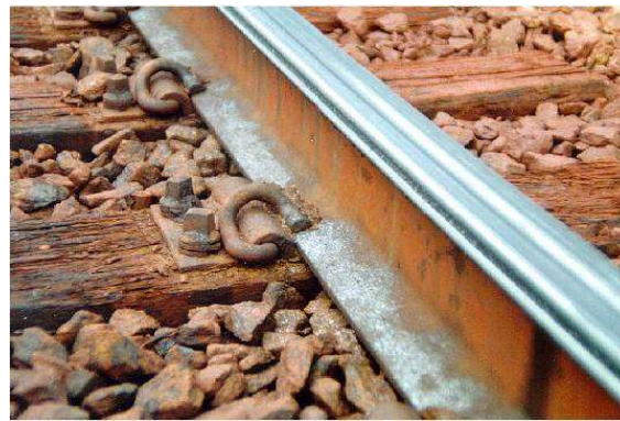
Rail wear, RCF, and spalling
