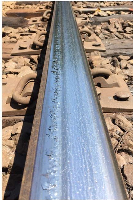
Rail wear, RCF, and spalling
