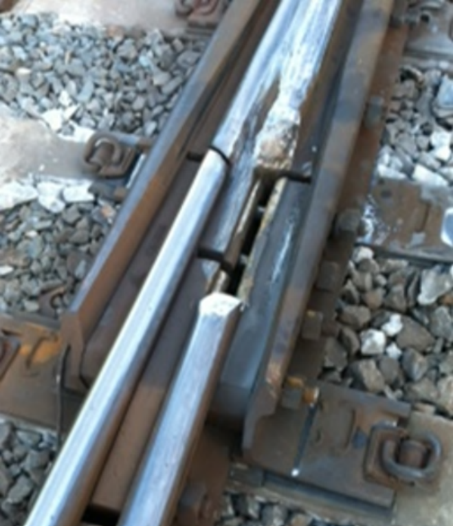
Cracked/Broken Frog
