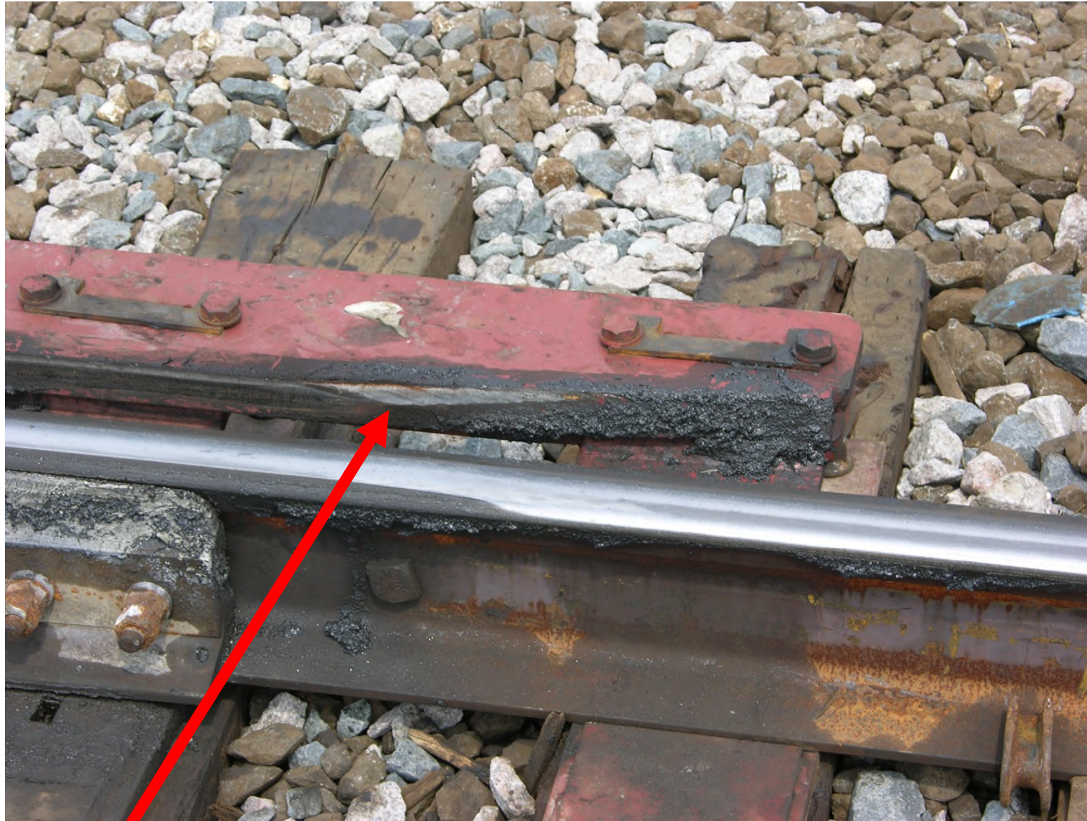
Heavy wear on switch point protector
