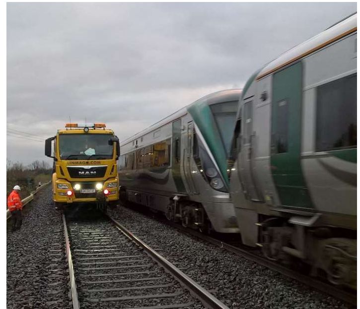
Milling machine working under single line possession
