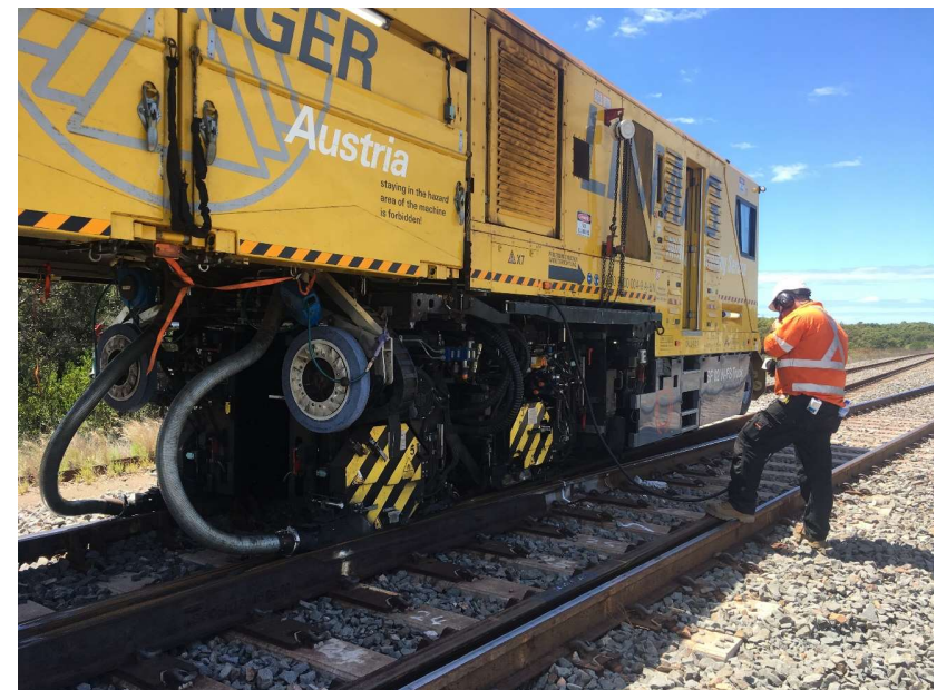
Example of switch treatment in Australia
