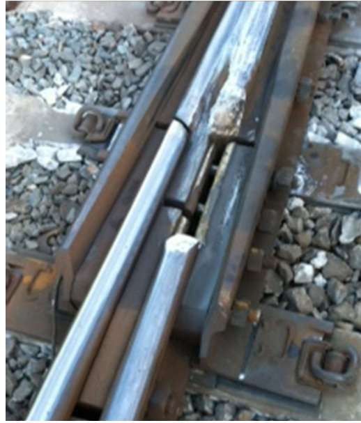
Cracked/Broken Frog
