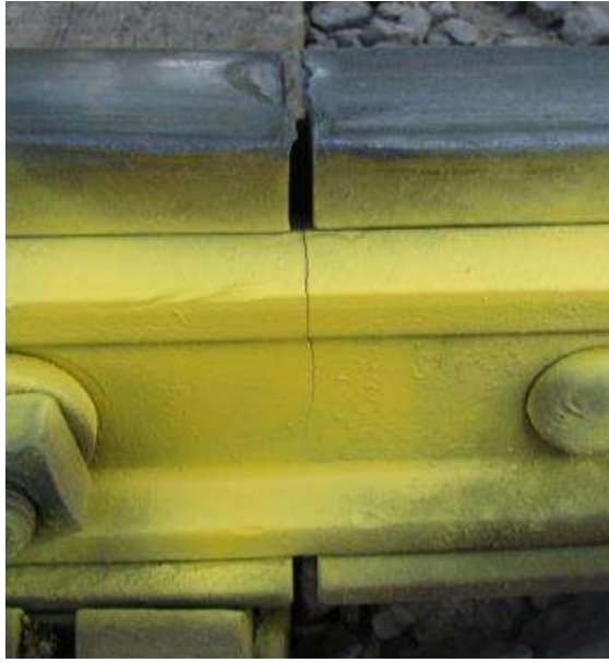
Cracked/Broken Joint Bar
