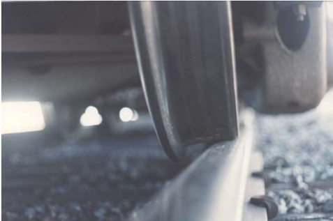
Field side contact low rail
